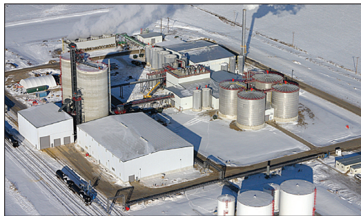
Golden Grain Energy LLC 40-million-gallon ethanol plant in Mason City, IA.
